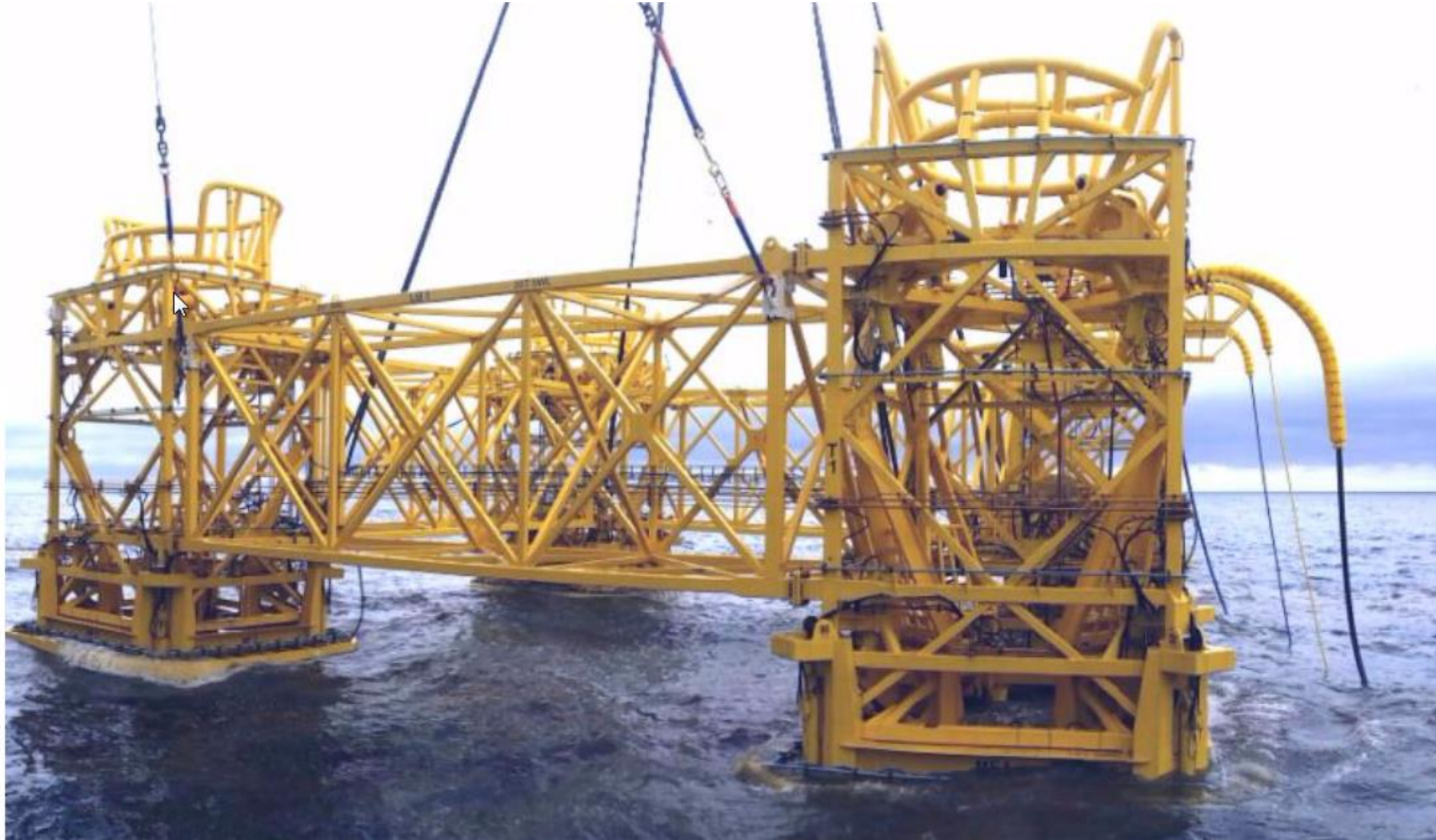
World's largest subsea piling template @ 20*20m
