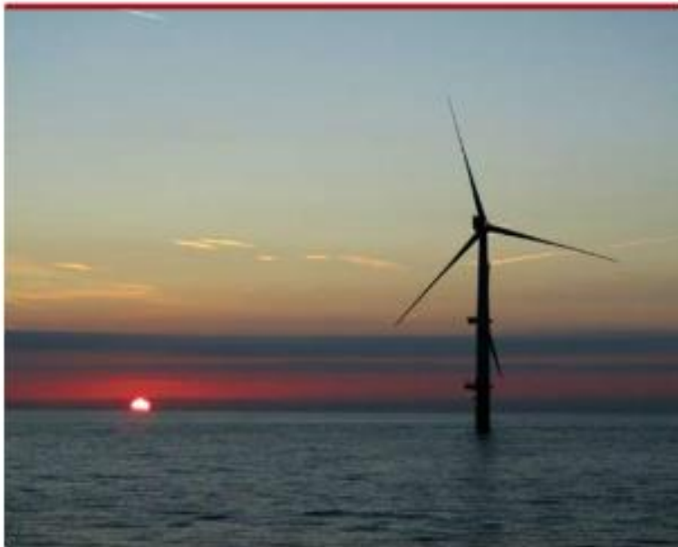
DEAD IN THE WATER: winter weather is holding up export cable repairs at Dong's Walney 2 wind farm in the Irish Sea
