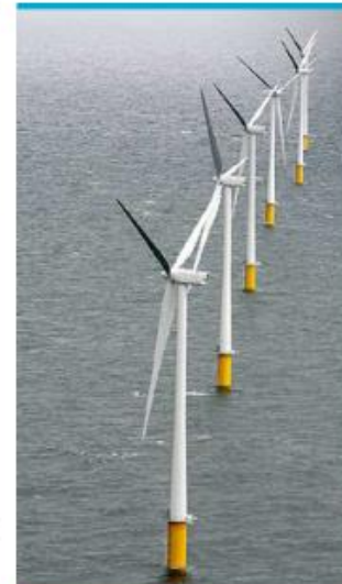
ROBIN RIGG: and then there was 174MW... Photo: Eon
